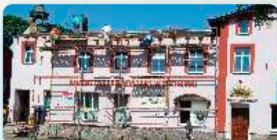
Remont dachu na GOK w Tuchomiu
